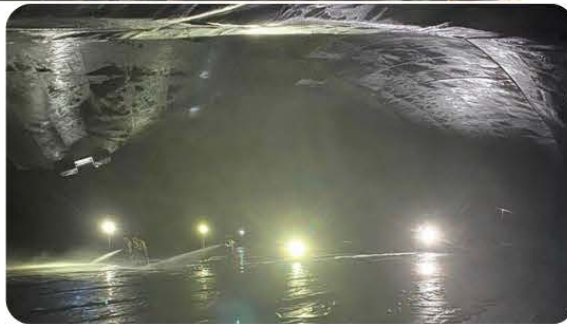
Immediate Left: Staff Washing and Inspecting Interior Reservoir Cover
