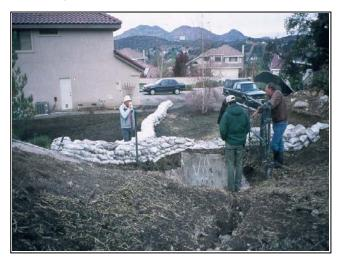
**Sandbags** are constructed of plastic, geo-textile bags filled with sand. A sand bag barrier is a temporary linear sediment barrier consisting of stacked sandbags designed to intercept and divert flow away from property and roads.
