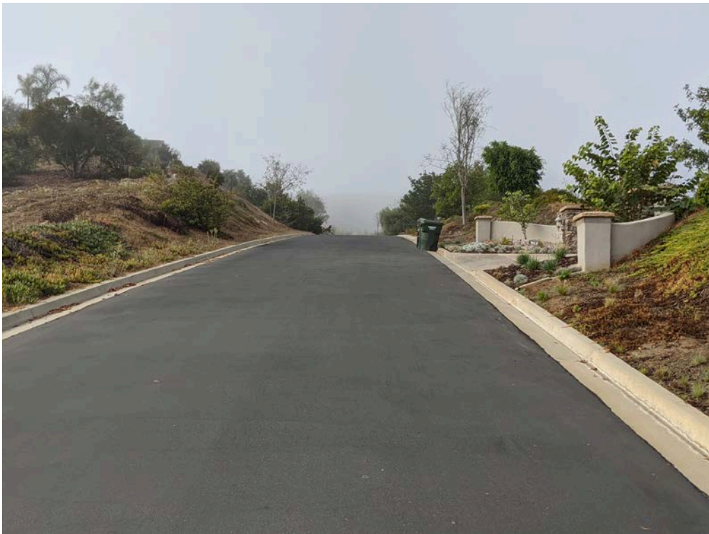
Northern end of Integrity Court looking south.
