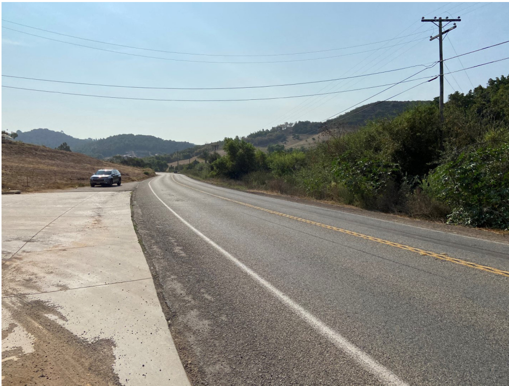
Western end of Gopher Canyon Road (Section 1) looking east.
