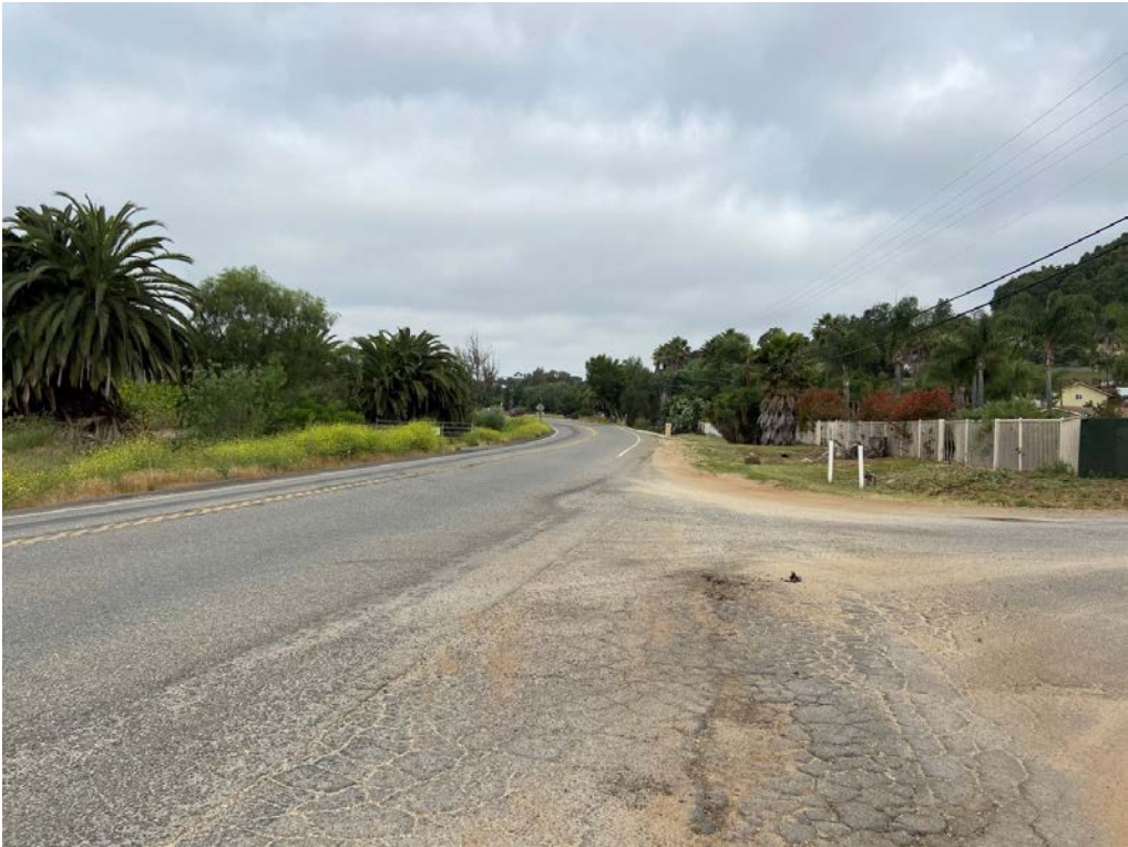
Eastern end of Disney Lane looking west.
