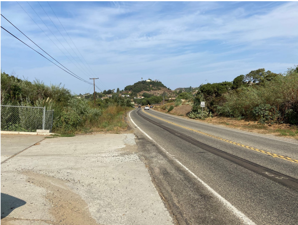
Eastern end of Gopher Canyon Road (Section 1) looking west.
