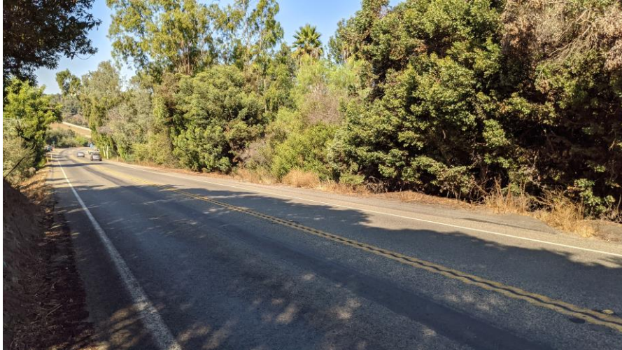
Plate 5. Overview of project alignment between Avohill Drive and El Paseo, view to the northwest.
