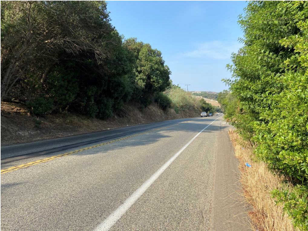
Eastern end of Gopher Canyon Road (Section 2) looking west.
