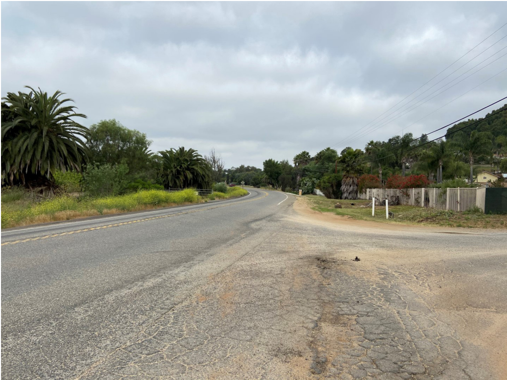
Eastern end of Disney Lane looking west.
