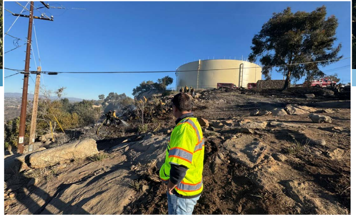
Rainbow Water General Manager, Jake Wiley assesses the Lilac Fire damage around Hutton Tank in Bonsall.
