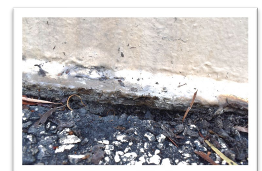
Tank Chime (deterioration)
