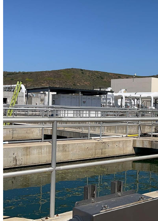
Skinner Treatment Plant, Temecula
