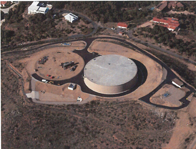
Pala Mesa Tank Site and 6 MG Storage Tank Project
