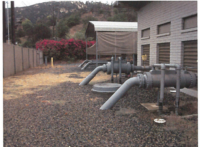
Pump Station #1 Natural Gas Motor Replacements
