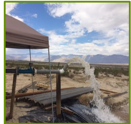
Well Development for new Water Supply
