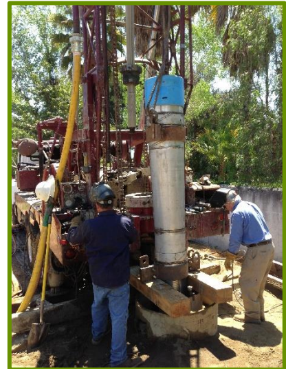
RPMWC Well 40 Casing Installation
