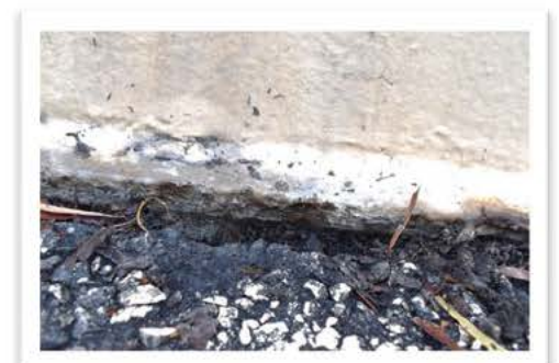
Tank Chime (deterioration)
