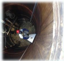
Our Wastewater staff also perform monthly manhole inspections to circumvent problematic situations such as roots infiltration, Fat, Oil and Grease (FOG) buildup, vandalism, and odor problems. They similarly perform maintenance and monitoring of all our smart cover units which are preventative measurement tools used to alert our staff when sewage is backing up so we can respond promptly.
