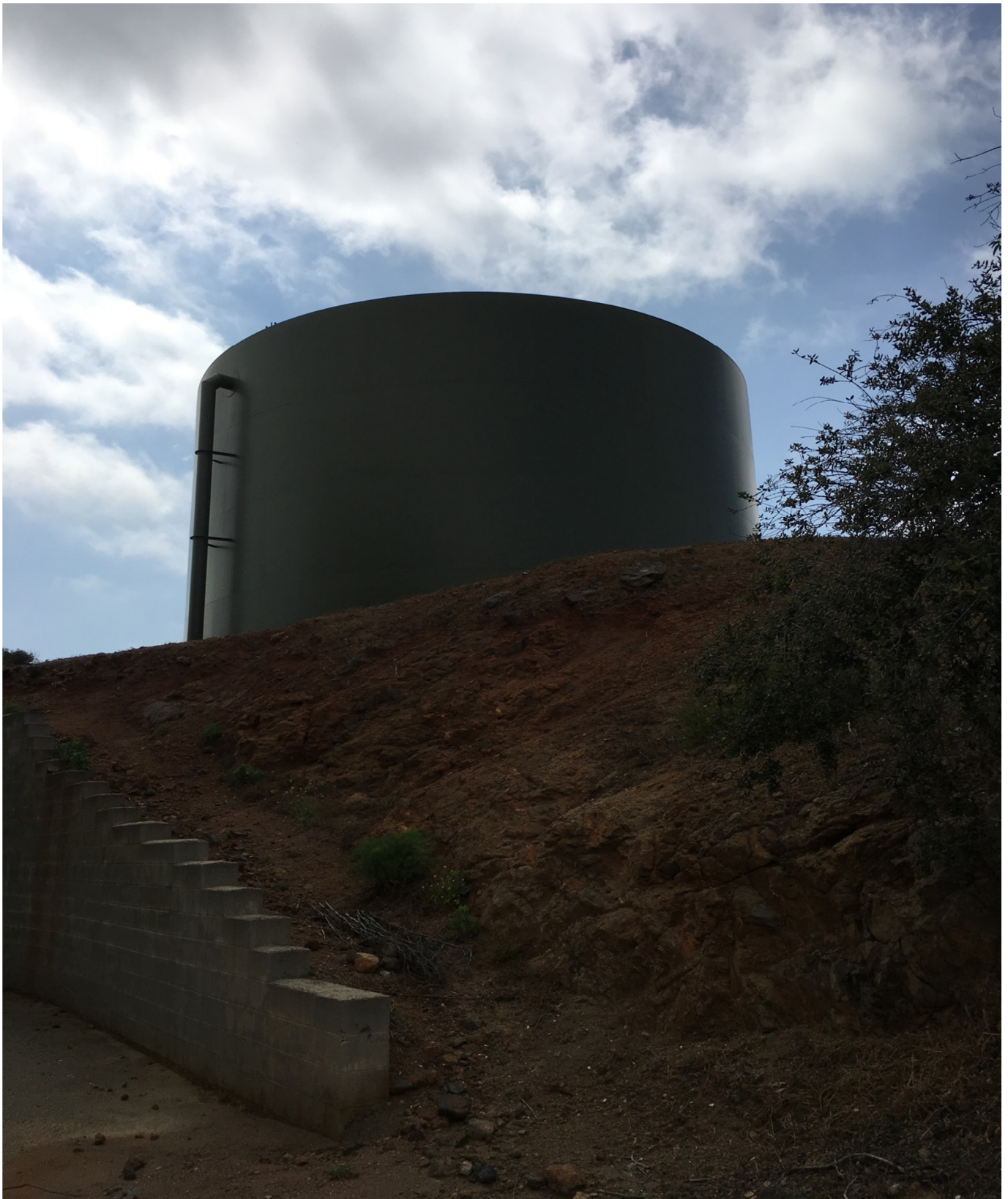
U 1 Storage Tank #1
