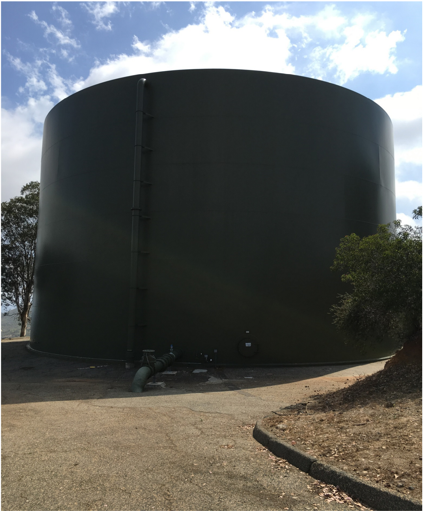
U 1 Storage Tank #2
