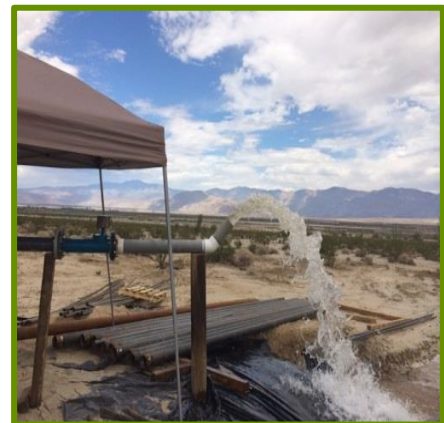
Well Development for new Water Supply
