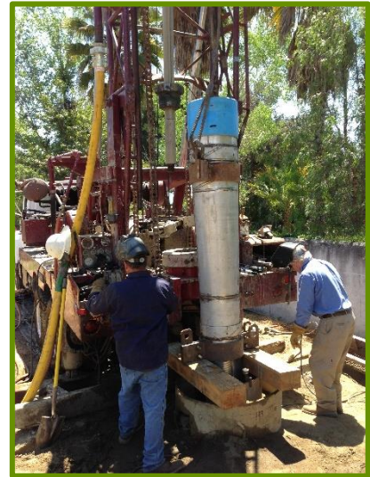
RPMWC Well 40 Casing Installation
